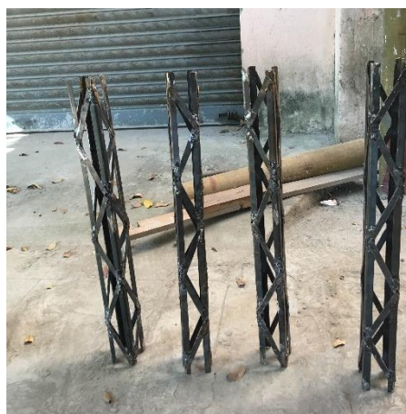
Figure 3. Reinforcement skeleton with Laced Configuration.
