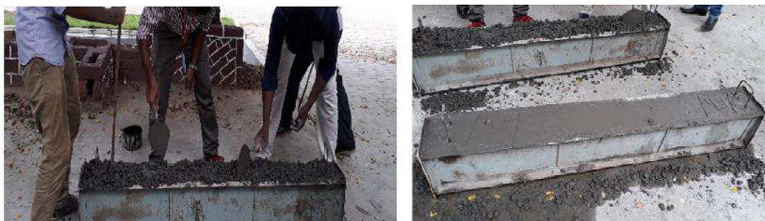
Figure 4 During and after casting of beams
